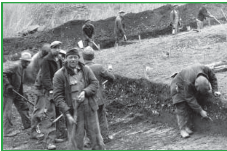
It's all in a day's work at this Muhlenberg County site: digging out the dirt and cleaning up the trench walls.
